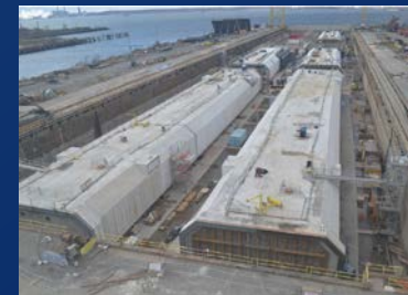
d) Immersed Tube (in dry dock)
