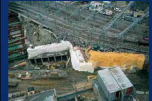
c) Jacked Tunnel
