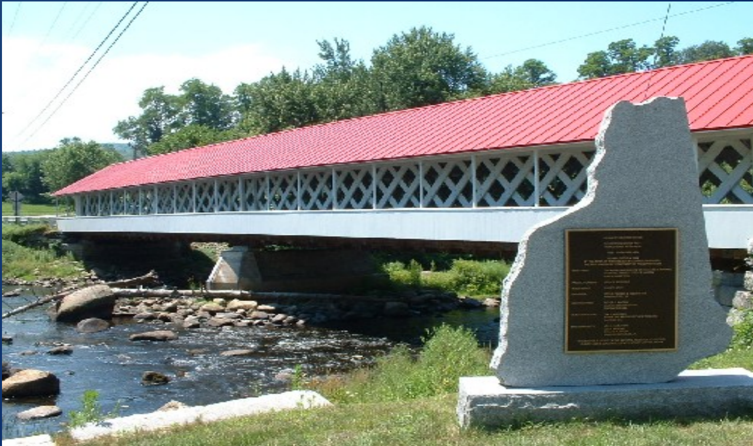
Ashuelot Covered Bridge
